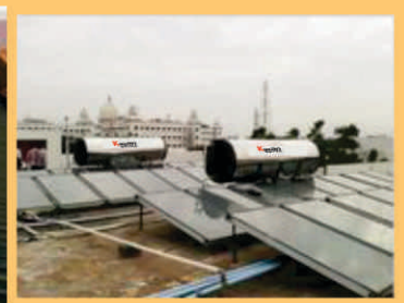
Capacity 5000 LPD (2500x2 No's) Economic & HR (Vent Type) Deluxe & HR (Vent Type), Hi-Tech & Hr (non-vent)
